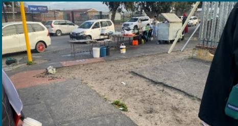
Nyanga: Sithandathu Ave - sidewalk not repaired and made good after underground trenching works
