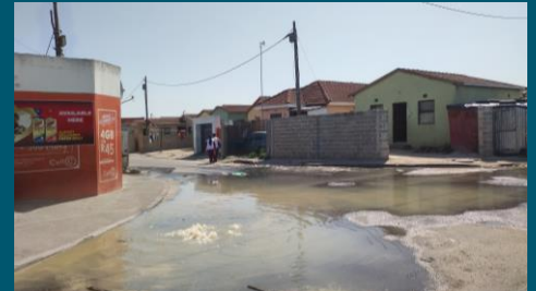
Near Nolungile PTI Precinct - leaking sewer main
