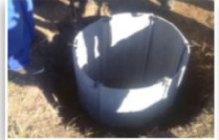
Precast concrete leach pit circular
