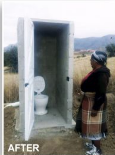
Upgrading of existing concrete block structure from VIP to Eaziflush – including new polymer door
