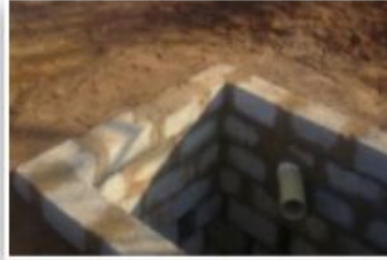
Standard M6 concrete block Leach pit
