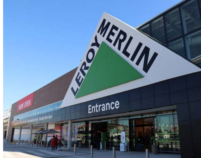
Leroy Merlin Little Falls Roodepoort South Africa
